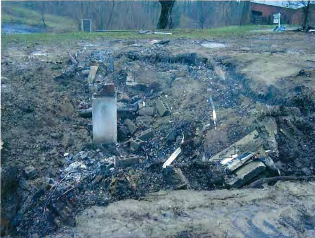
Date: 1/10/2008 Time: 12:44 P.M. Direction: southeast Photo by: S. Williams Exposure #: 003 Comments: metal, demolition wood, brick, concrete & ash
